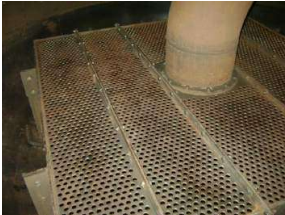
Perforated plate in D70702 looseness
